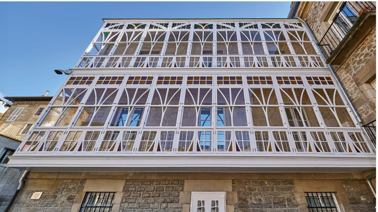
An added complexity was the different window shapes, sizes and patterns, which required precision design planning and documentation. Each glass element needed dismantling, numbering, and analysis to identify damage and ensure accurate restoration.
