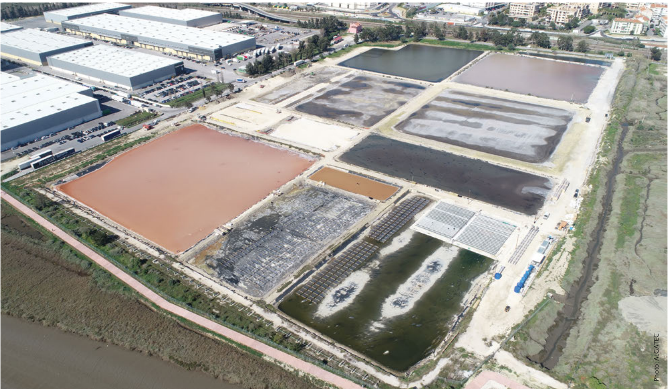
Aerial view of ALGATEC Eco Business Park production site. Under construction in Póvoa de Santa Iria (15 km northeast of Lisbon), this will be the largest microalgae production platform in Europe (14 ha). An Eco Business Park designed to welcome companies and entrepreneurial projects in the field of sustainable algae business.
