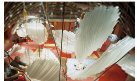
The installation of the sculpture took two months. 600 steel cables allow the glass clouds to float in the atrium of the DG Bank. The suspension construction is designed to support 14 times the actual weight of the pieces.
