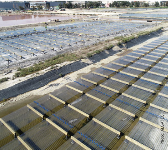
In the microalgae production systems at the ALGATEC Eco Business Park, A4F also uses tubular glass photobioreactors.
