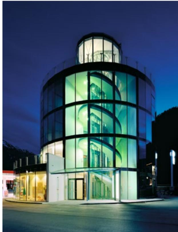
A frameless, point-supported glass facade was created for the **Bluetower in St. Johann** with SCHOTT fire resistant glazing. The connection of the double-glazed elements with PYRAN® S was achieved using purpose-built steel sections, which were attached with stainless steel point fittings at each intermediate floor.
