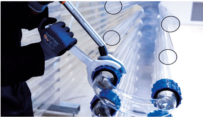
10 Next push the U-Bend over two tube ends at the same time. Afterwards tighten the blue nuts as shown, before the U-Bend is fully mounted to the system.
