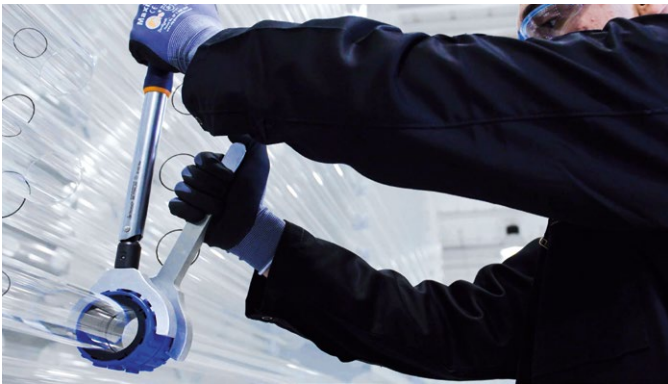
8 Now turn the wrenches in opposing directions until the torque wrench tilts towards your body. The connection process is now completed.
