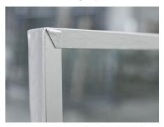
PYRANOVA® with intact edge protection sealing tape (silver)
