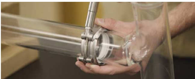
Joining KIMAX® Pipe with bead-to-plain end coupling.
